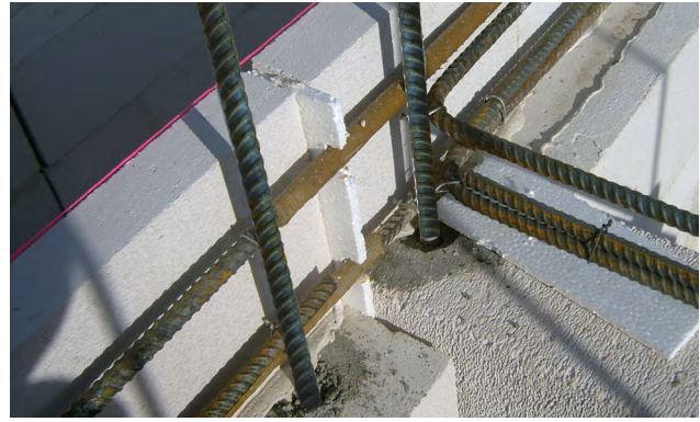
Movement Control Joint under Construction
