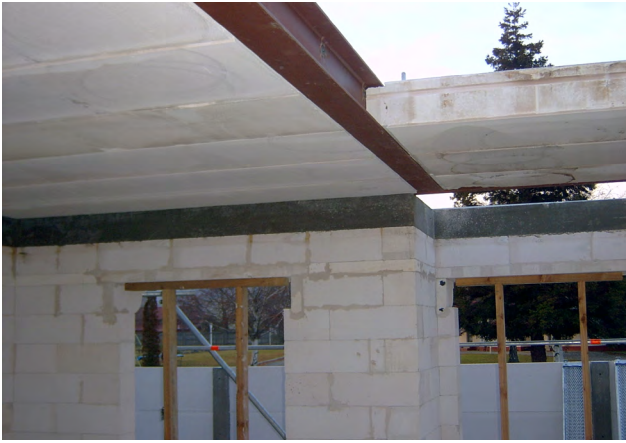
Underneath floor panels showing poured concrete of bond beam on panel side.
