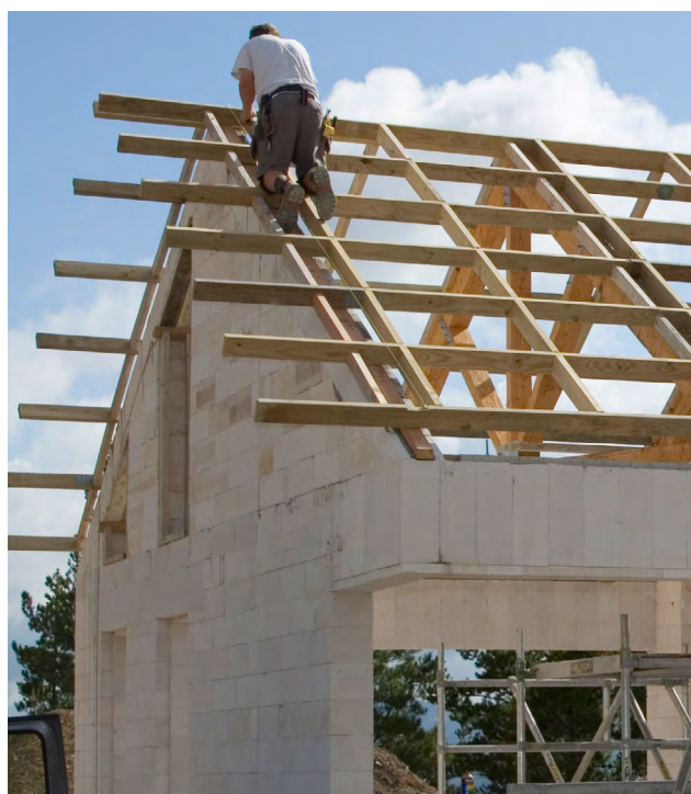
Raking bond beam
