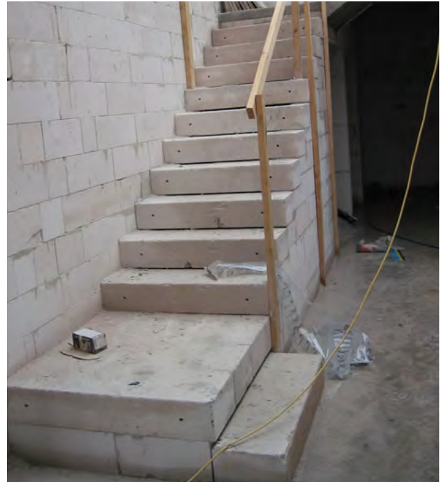
Stairs under construction in block wall
