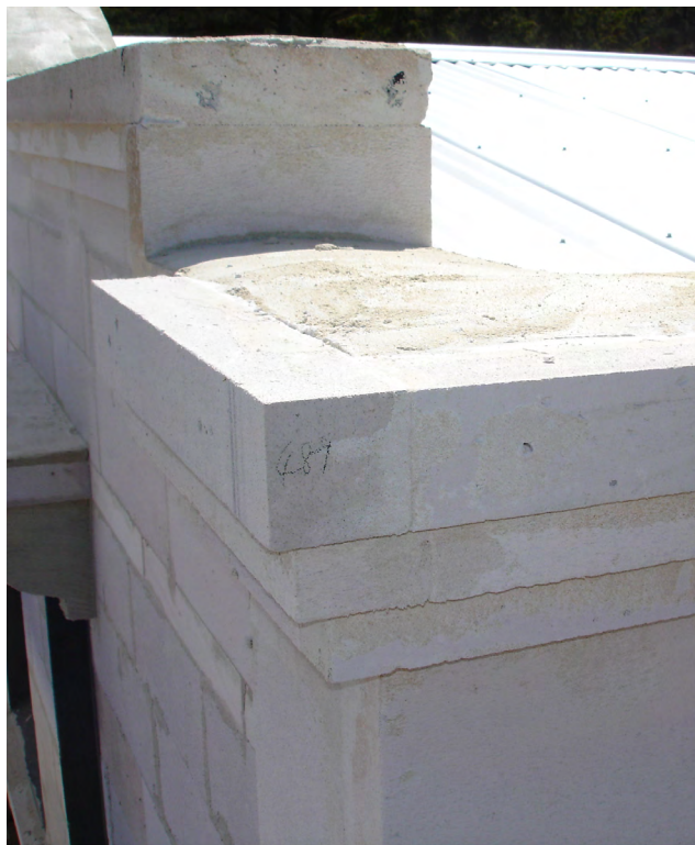
Photo of panel being glued to block wall as mouldings
