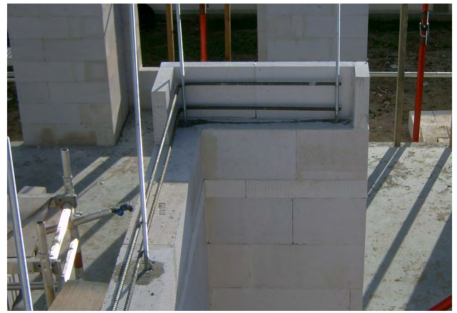
Bond beam reinforcing with facing blocks being fixed into place.
